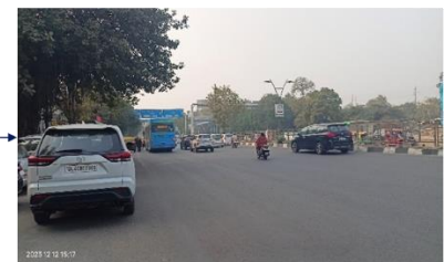
Absence of road markings, signage and speed control measures at the intersection.
