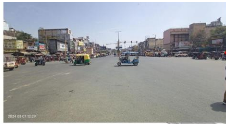
Wide open junction , absence of channelisers
