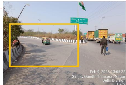
Larger turning radius provokes speeding at each arm.
