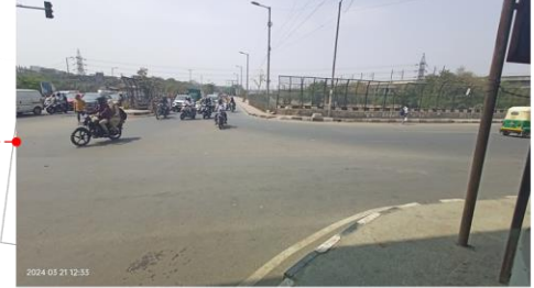
Absence of zebra crossing, kerb ramp and bollards at junction
