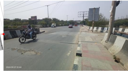
Damaged & uneven road surface and pedestrian infrastructure
