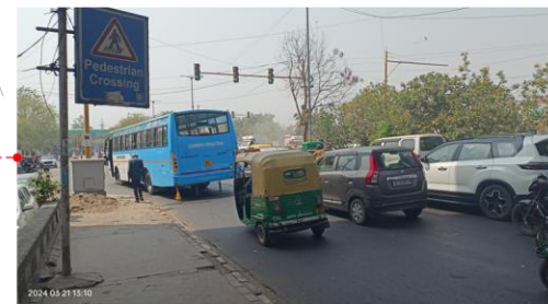
Absence of kerb ramp and bollards at junction
