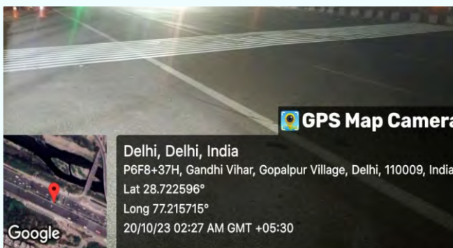
Traffic Calming Measure: Rumble strips; Road Marking: Chequered Box
